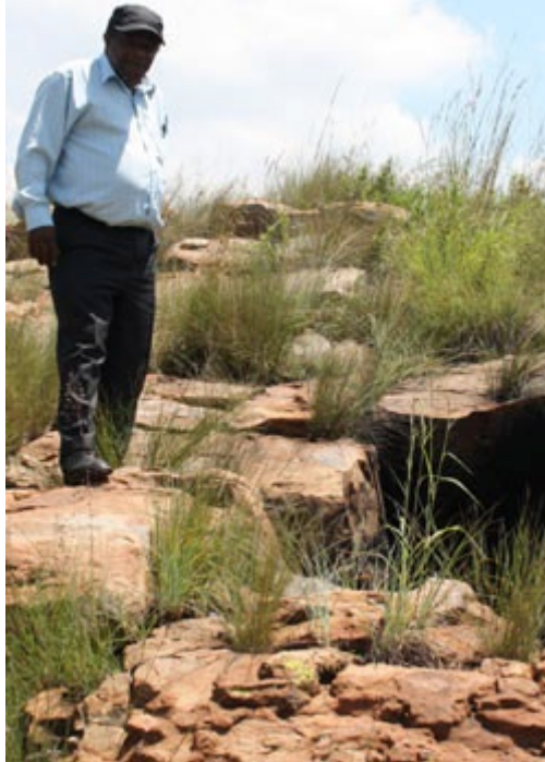
Adam Mathysen standing alongside one of the four disused mine tunnels along the banks of the Klip River
